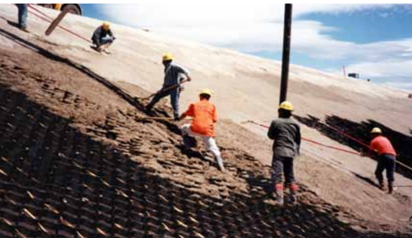
5. Concrete Placement with Pump
