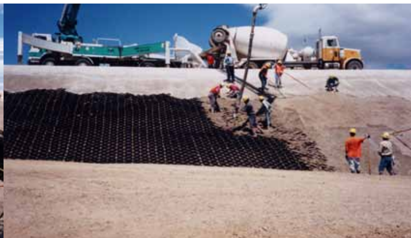
6. Concrete Placement with Pump
