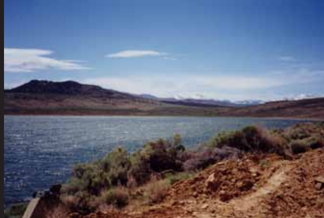
1. View of reservoir from crest of old dam
